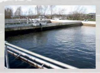
Scottish Water were required to upgrade the Sterling Wastewater Treatment Plant to improve the quality of the effluent in line with the European Urban Wastewater Treatment Directive (UWwTD). The upgrade included the removal of ammonia from the effluent that the
